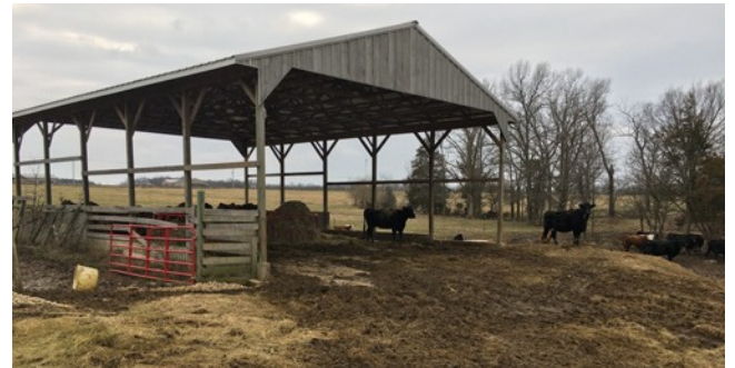
N312 Beef and Small Ruminant Waste Management: Winter Feeding Facility
