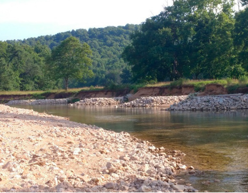
C650 Streambank Stabilization
