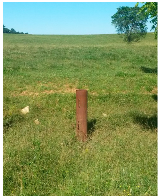
DSP-31 Sinkhole Improvement: Vertical Drain
