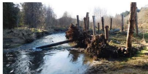
Instream and streambank stabilization structures: Benefits include erosion control and enhanced fish habitat.
