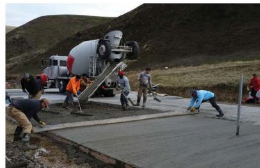
Livestock feeding pads and heavy use areas: Installing stable, non-eroding surfaces in areas frequently used by animals prevents erosion and aids in manure collection. This helps protect water and air quality.
