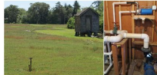
Chemigation units: This upgrades irrigation systems to allow for more efficient application of chemicals to cranberry bogs and reduces runoff to shellfish growing areas.
