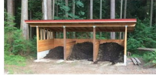
Waste storage facilities: Storing manure in a covered structure on a non-erodible surface reduces the potential of polluting surface and groundwater.
