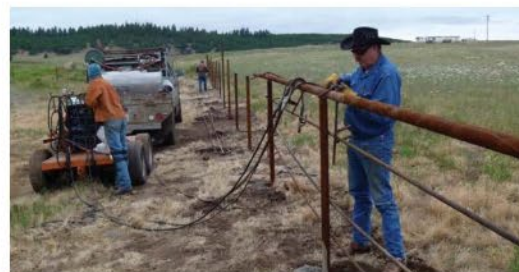
Fencing and livestock exclusion: This helps prevent animals from accessing streams and other critical areas and can improve pasture quality.
