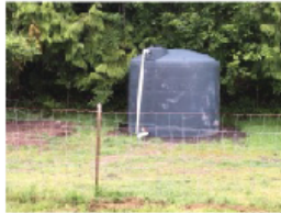
Stormwater management and livestock watering tank for a sheep operation improving water quality in Discovery Bay
