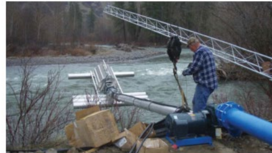
Fish screens: These are required on IEGP projects. They protect juvenile fish from water diversions, such as irrigation pump intakes.
