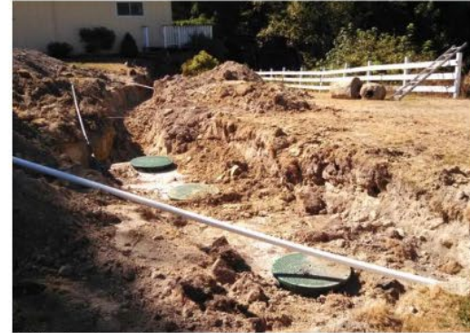
On-site septic system repair or replacement: Failing septic systems have proven to be a significant source of water pollution in some shellfish growing areas.
