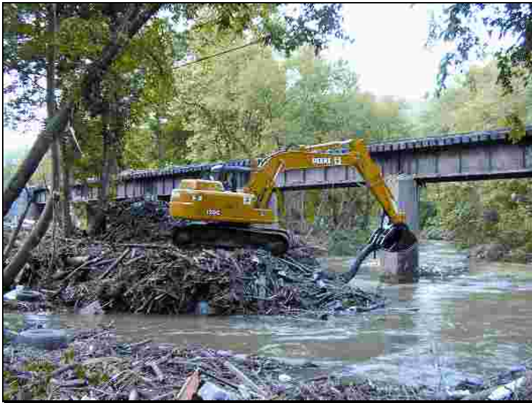
This contractor at Pigeon Creek worked quickly to remove a hazardous stream debris blockage near a railroad trestle at Belo in Mingo County in August 2004.
