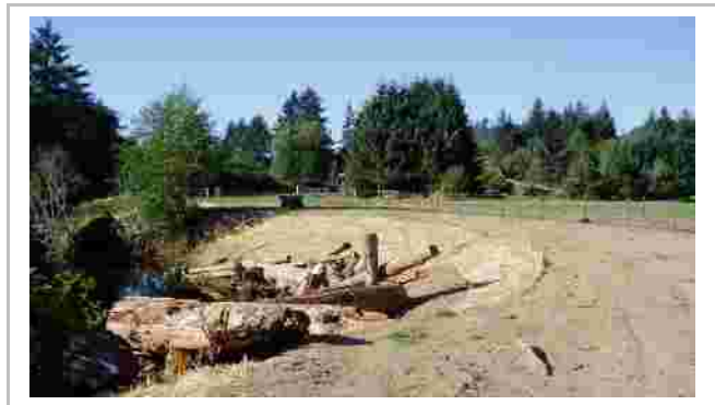
Clallam River Bank Stabilization at Sadilek Farm
