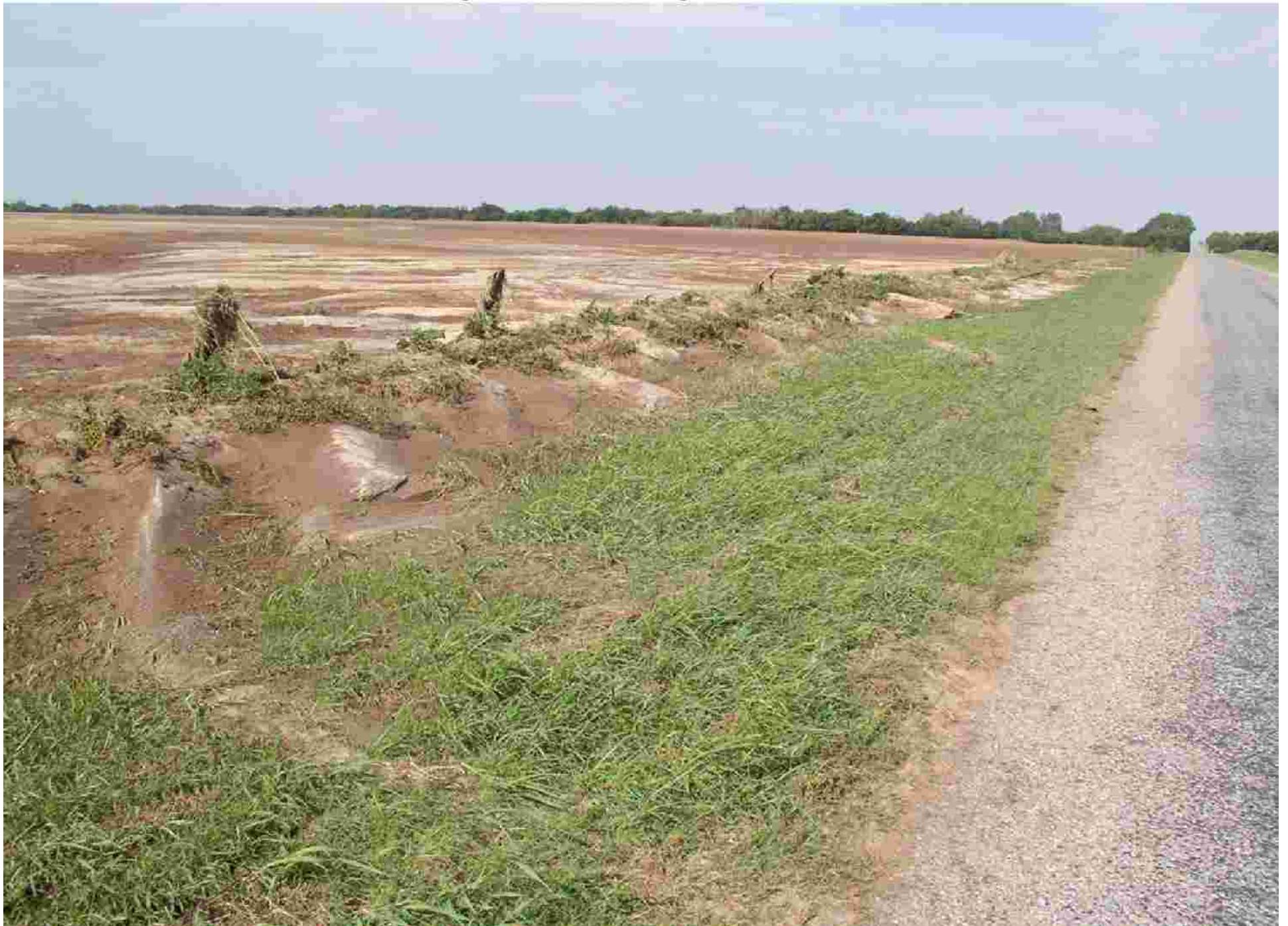
Kingfisher area flood damage
